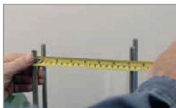
2. Measure the distance between the two V-brackets
